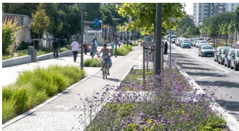
Requalification de l'avenue Mermoz, France
